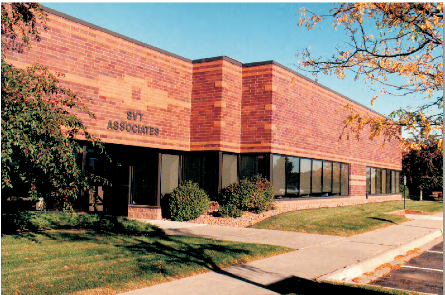
SVT Associates Manufacturing and Research Facility in Eden Prairie, MN
